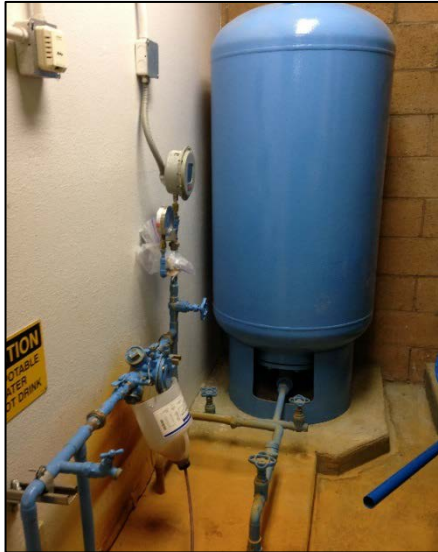
Photo 11 – Hydropneumatic Tank
