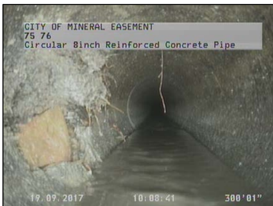
Photo 15 – CCTV Showing Root Intrusion
