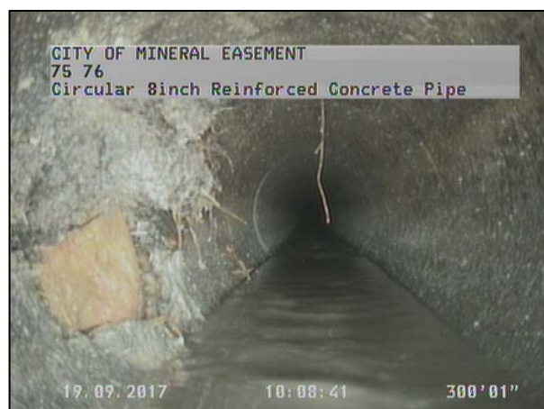
Photo 15 – CCTV Showing Root Intrusion
