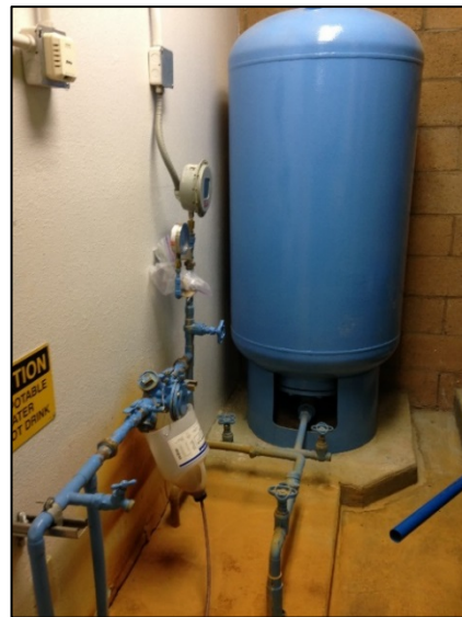
Photo 11 – Hydropneumatic Tank
