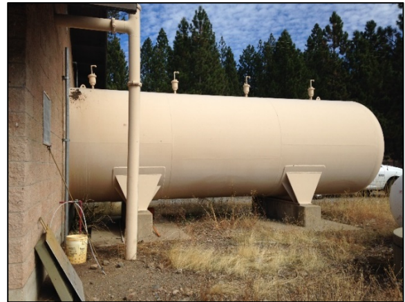
Photo 8 – Pressure Filter
